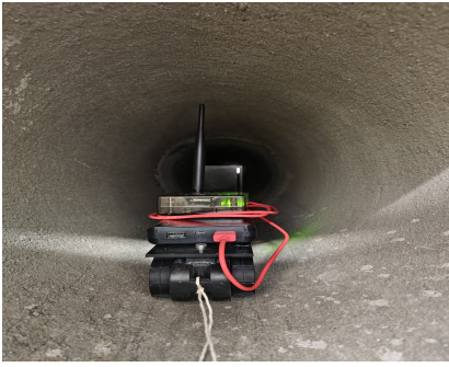
(a) The S node placed inside the buried concrete pipe of diameter 300 mm.
