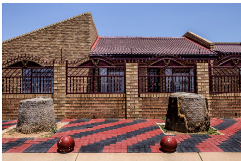
Figure 6.3 Housing improvements in Ekangala (source: Mark Lewis)
