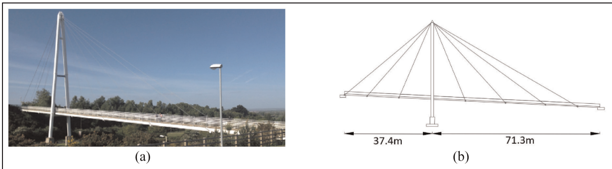
Figure 13. (a) A photograph of the cable-stayed bridge. (b) A schematic of the bridge.
