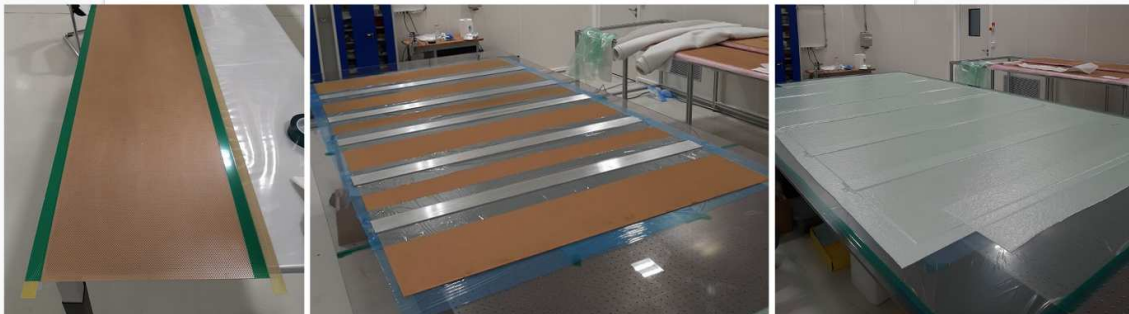
Figure 3.34. Left: preparation of PCB segment for epoxy application. Middle: six PCB segments are glued, aligned and ready to be sealed. Right: glued assembly is under vacuum for drying.
