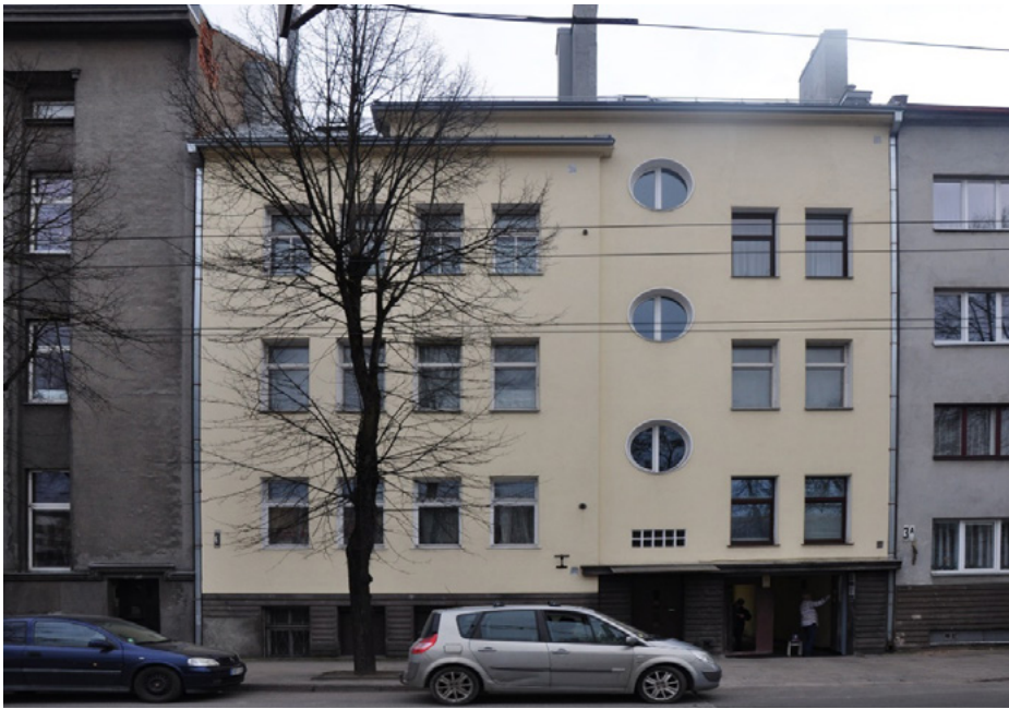
Fig. 4. The building at Kęstučio Street, 3, which was demonstrated in the experiment
