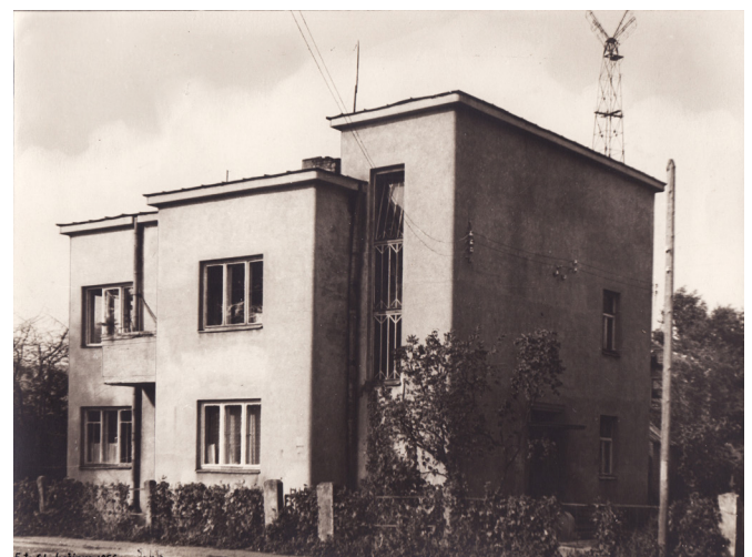
Fig. 6. Imitated flat roofed house in Žaliakalnis district [KTU ASI archive, photograph by S. Lukošius].
