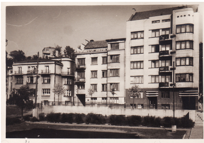
Fig. 8. Apartment buildings in Kaunas city centre [KTU ASI archive, photograph by J. Skeivys].
