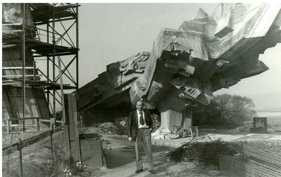
Figure 4. Architect V. Vielius during the process of the construction of the Ninth Fort monument in Kaunas, the late 1970s. From the Kaunas Ninth Fort museum.
