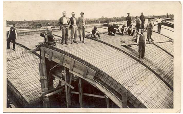
Figure 1. Construction of the factory buildings (source: Bayındır, 2019)
