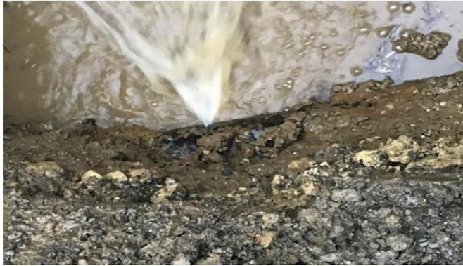
Figure 1: Example of a leaking cast iron pipe from Barton et al. [1].
