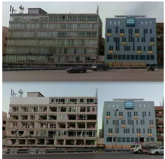
Figure 6 Different damage observed for different glazing systems at Location 2; before [top] and after [bottom] the explosion [3]
