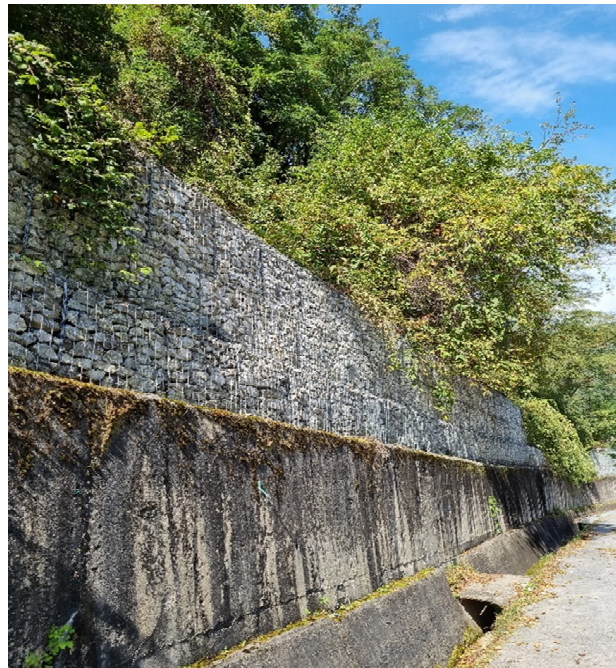
Figure 8. Complex GGSJ (concrete, gabion, artificial soil).
