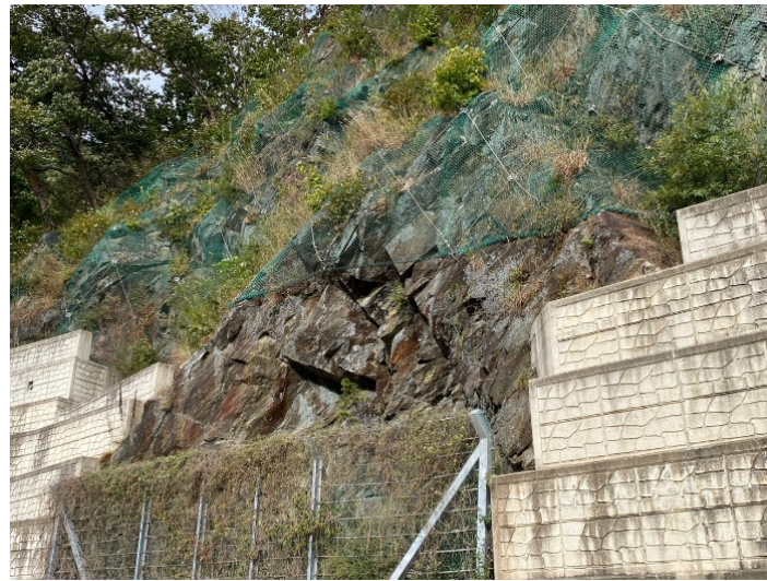
Figure 9. Complex GGSJ (artificial rock slope, concrete embankment).
