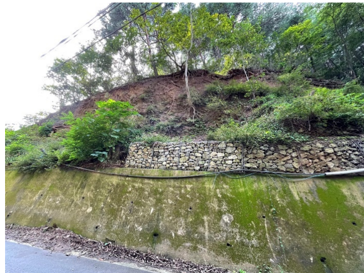
Figure 10. Complex GGSJ (artificial soil slope, artificial rock slope, gabion, concrete embankment).
