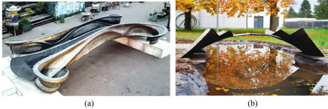
61 Figure. 1. 3D printed bridges: (a) a MX3D metal 3D printed footbridge [5], and (b) a small 3D printed 62 footbridge in shell form [6].
