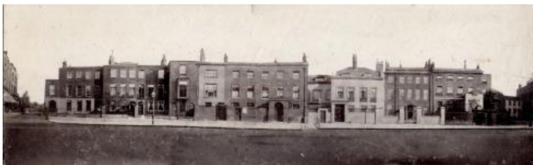
Figure 1: The Terrace shortly before its demolition in 1893 (Walker 2015).
