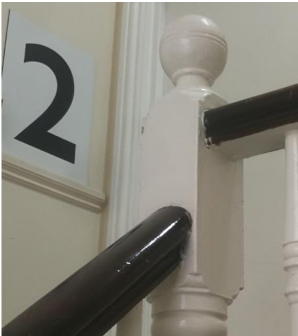
Figure 11: Floor number plastered in the building.
