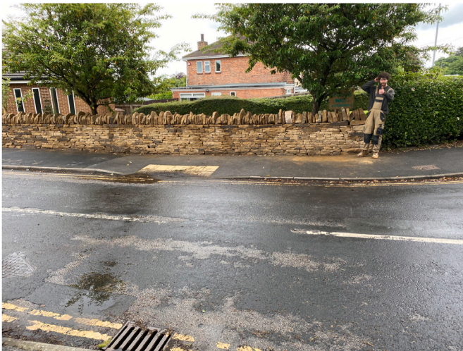
Fig. 6. The completed job.
