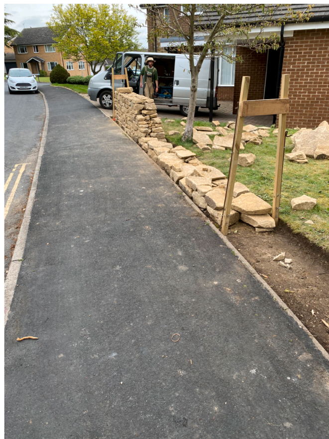
Fig. 4. Building the Wall in 6 m sections.
