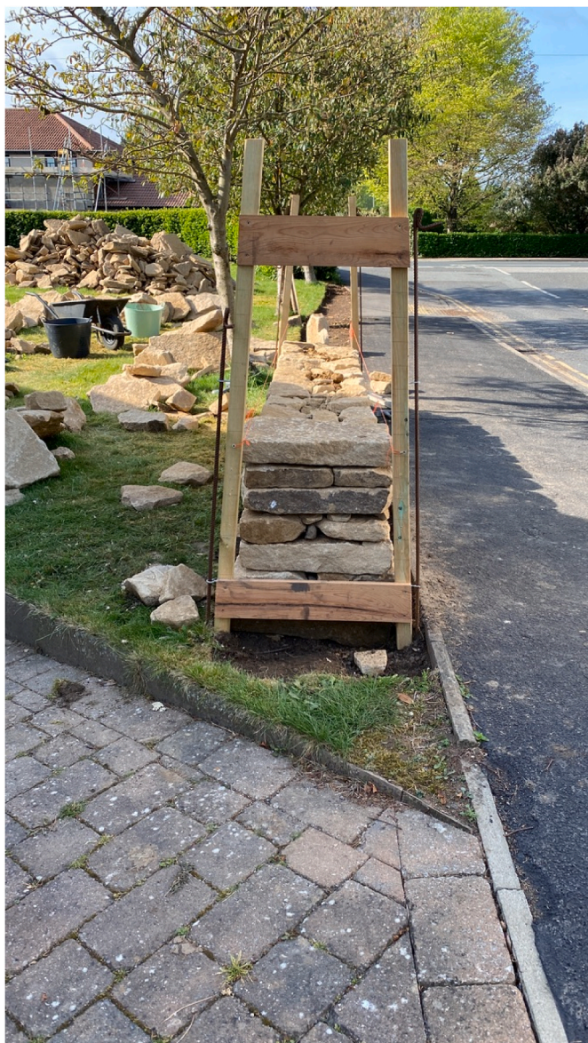
Fig. 3. Erection of batter boards.
