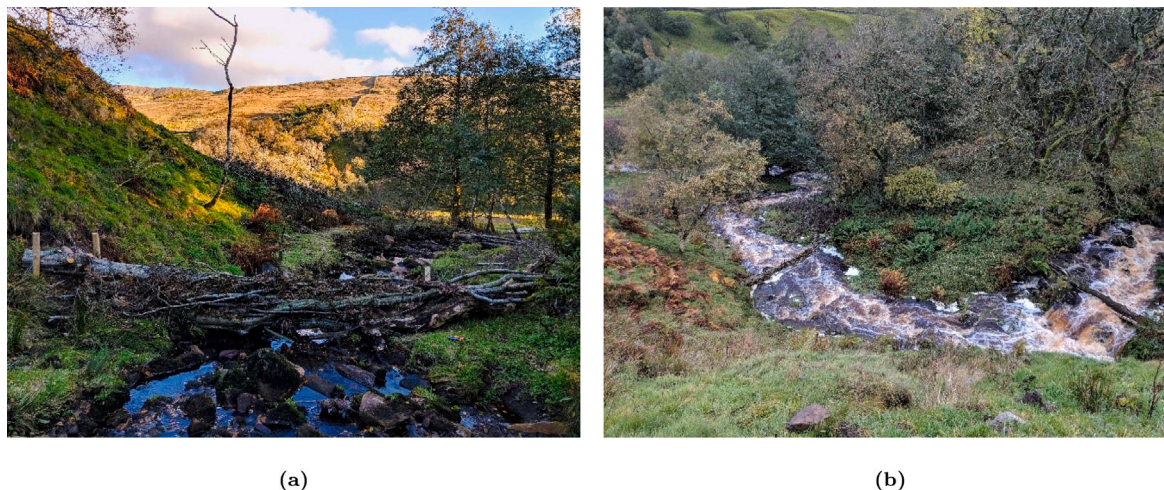
Fig. 2. Photographs of typical leaky dams on the impact stream: (a) elevation during baseflow conditions and (b) plan view during a high flow event.
