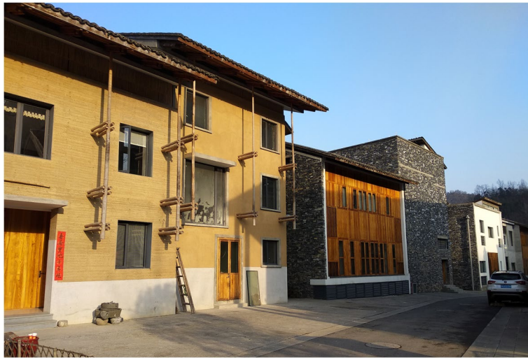
Fig. 7 The material tectonic of the vertical doorways, horizontal openings, wood shutters, deep eaves and shading devices (Source: the author)
