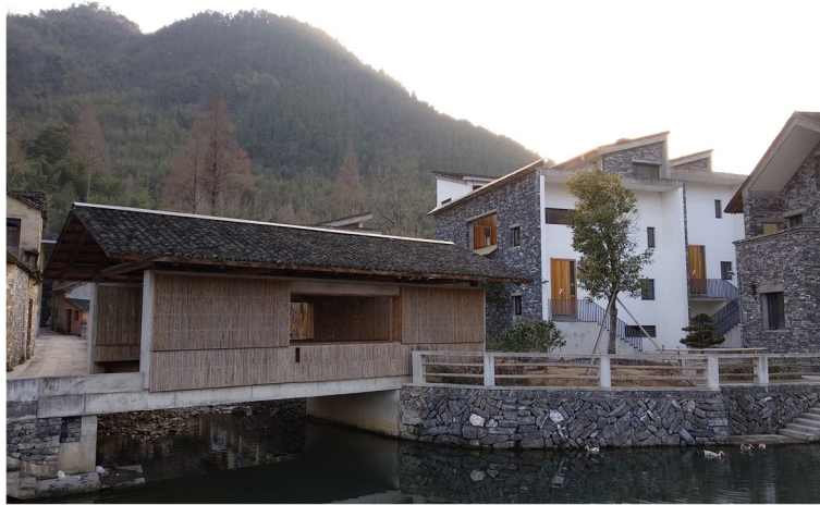
Fig. 4 The new wind-rain bridge with concrete load-bearing walls and wooden roof is placed at the intersection between the new and old villages, marking a communal focal point (Source: the author)
