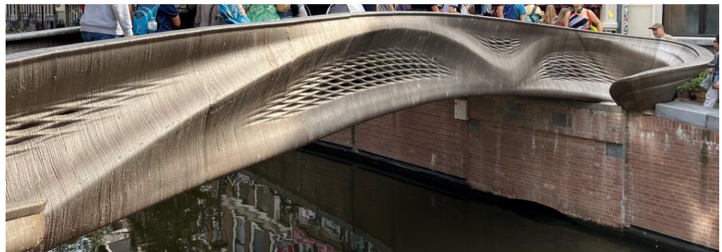
Figure 10. Additively Manufactured Bridge.
