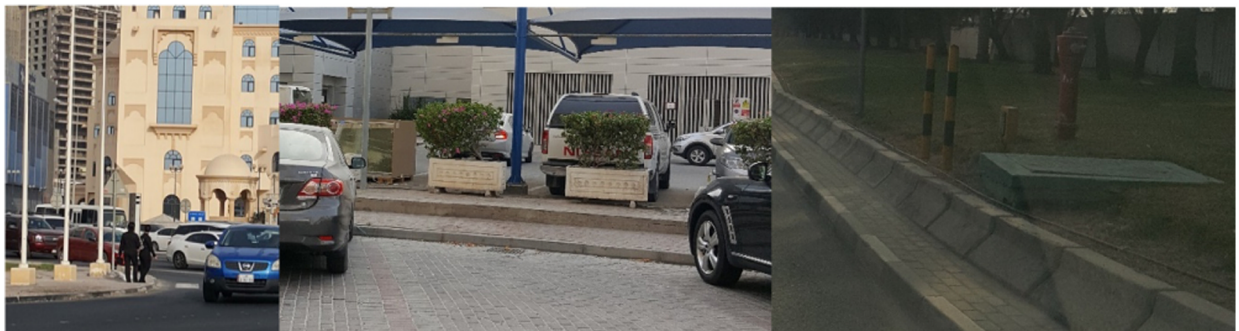
Fig. 18. Poor Pedestrian Walkways, Connectivity and Infrastructure (Source: authors).
