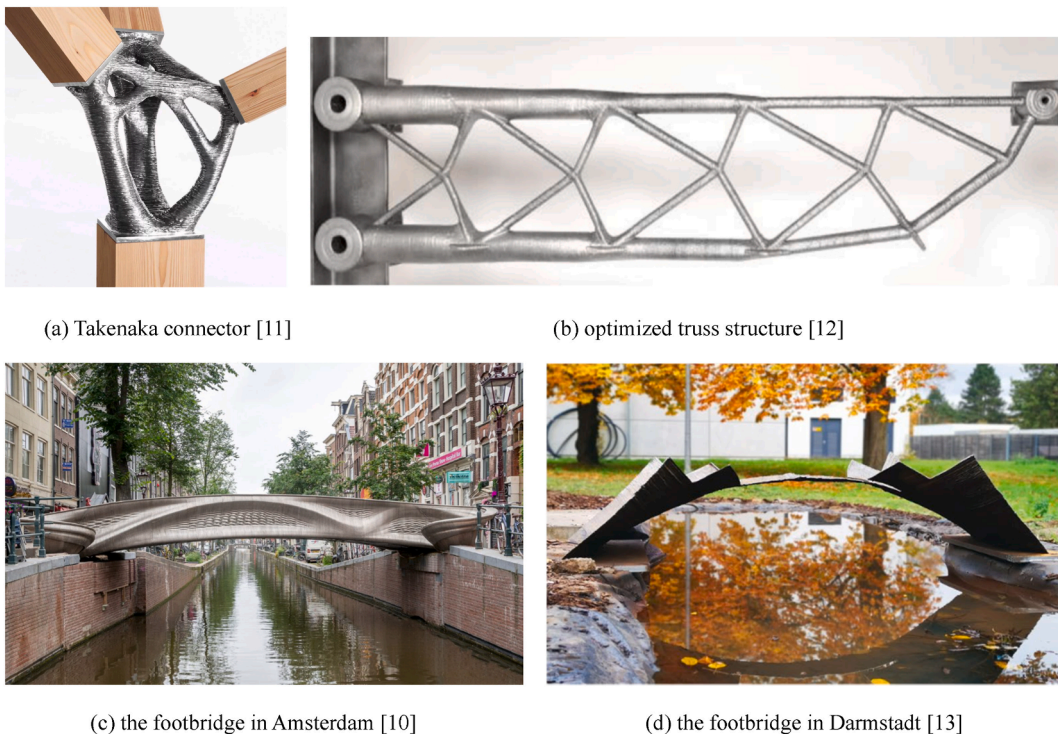
Fig. 1. WAAM structural components in the construction field.
