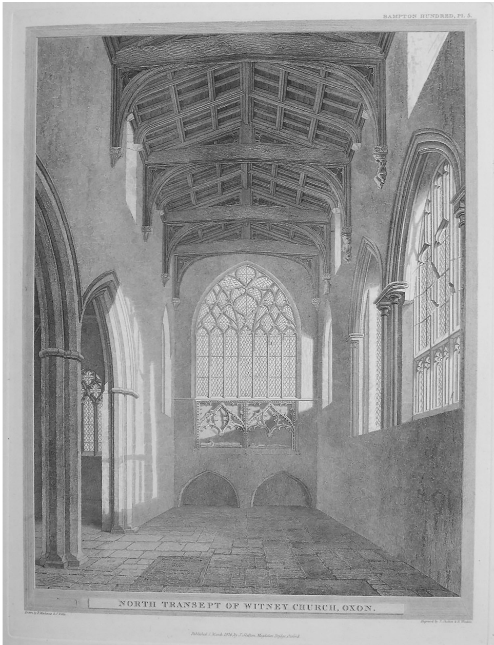
FIG. 8. Print of the interior of the north transept of St Mary, Witney (Oxfordshire), after an engraving by Joseph Skelton, c. 1823. This depicts the relieving arches for short light-shafts which illuminated the crypt below
