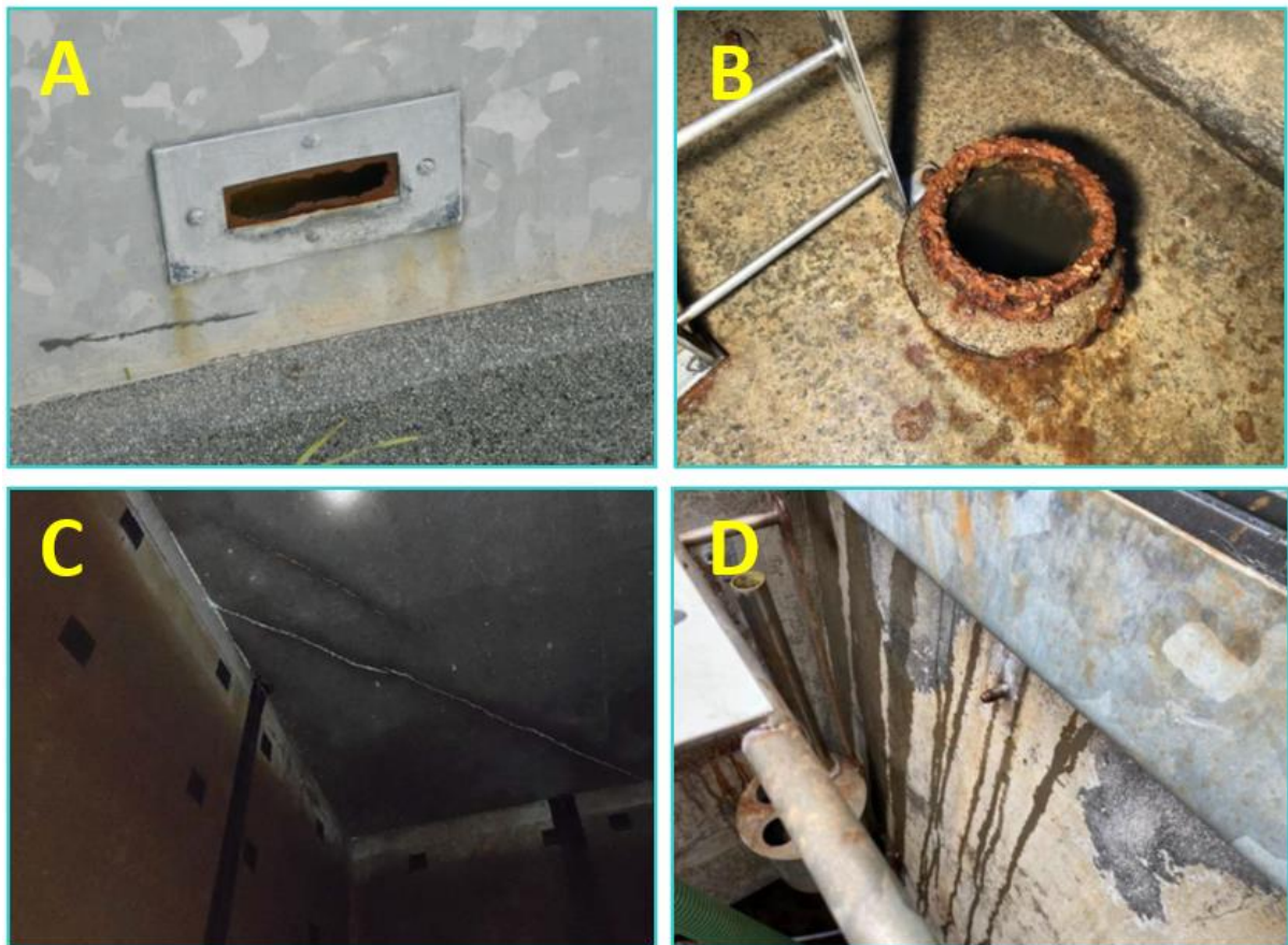
Figure 1 – A collection of photos showing some common issues seen in service reservoirs: A broken and corroded air vent (A), corrosion of internal structures (B), staining on walls and cracks in the roof (C), and ingress through the seam of an access hatch (D).
