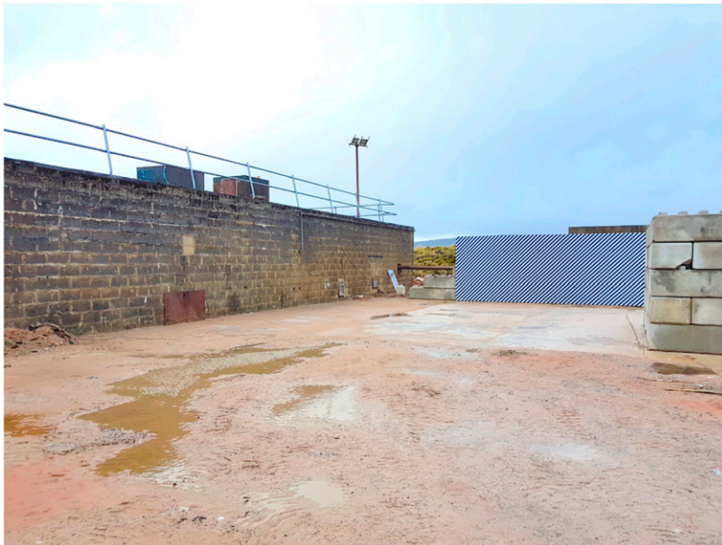
Figure 3. General arrangement of the test pad at the University of Sheffield Blast and Impact Laboratory: Site photograph taken approximately from the location of the high speed video camera.
