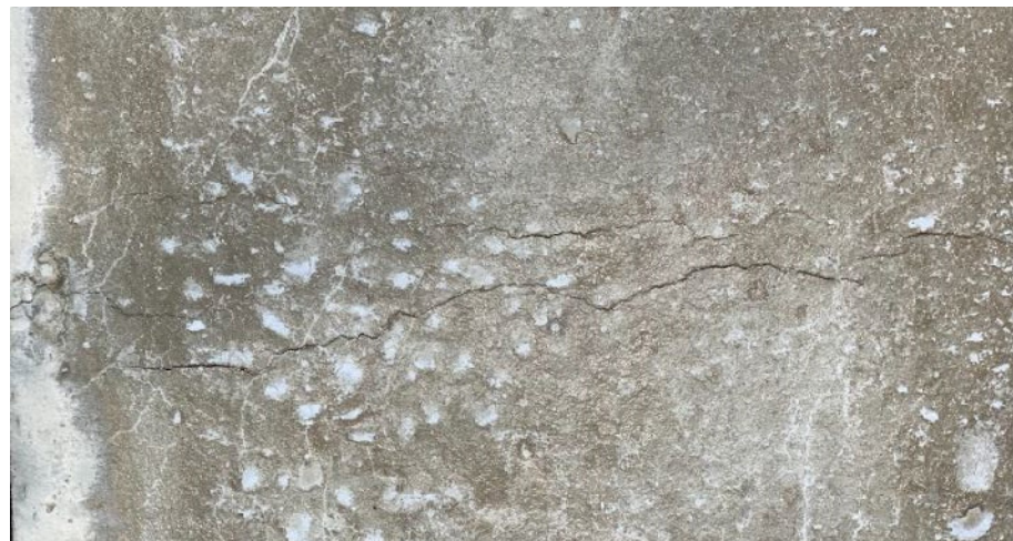
Figure 11. Typical crack pattern in plain concrete (PC) specimens of high temperature examined at 24 h.
