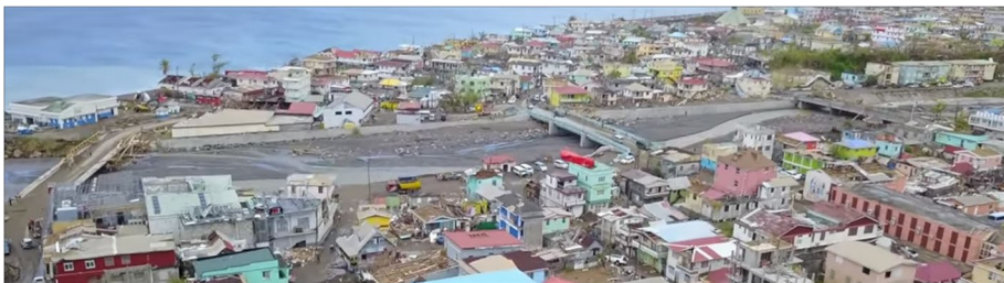
Fig. 5 Roseau Bridges 1, 2, 3 post Hurricane Maria. Left hand side of photo is downstream. Source: 4:03 min, https://www.youtube.com/watch?time_continue=8&v=_BIP5A3gT1o
