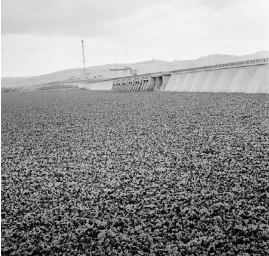
Inga-1 Hydro in its first year was already clogged by weeds. 1973, (Mieremet Rob / Anefo)
