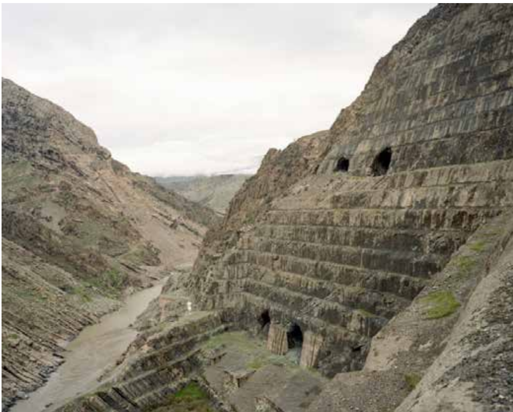
Bekhme dam, Bradost district, Iraq. 23 november 2018. ((C) Alex Kemman)
