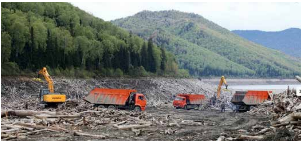
Scavenging floating wood from Sayano-Shushensky hydropower reservoir, Russia. (Rushydro)
