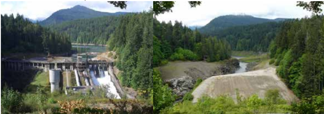
Left: Elwha Dam under deconstruction (Ben Cody/ Wikimedia), Right: Elwha Dam Finished, May 2013 ( Zandcee/ Wikimedia)
