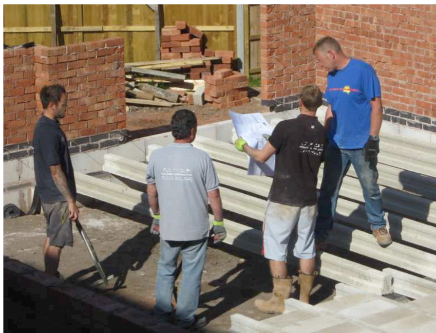
Photo 4.3: Operatives planning awkward lifts, regarding method as well as location (Photo Gibb).
