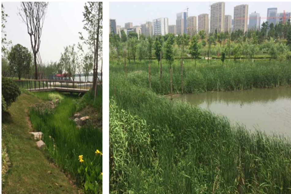
Figure 2 | SCP infrastructure in Jiangbei District, Ningbo. Bio-swale (left) and artificial wetland (right) (Source: Authors).
