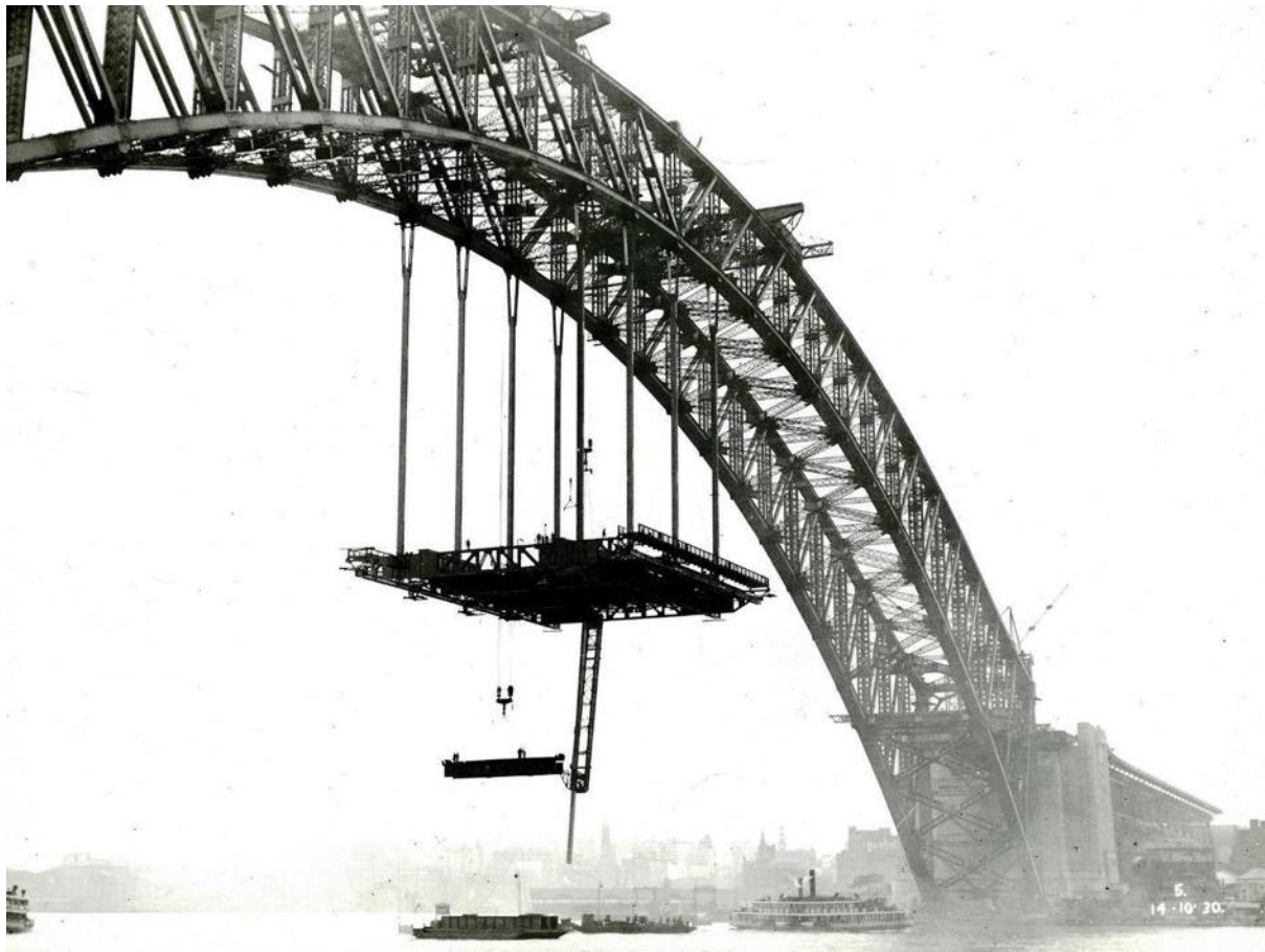
Construction of Sydney Harbour Bridge © Teesside Archives, Cleveland Bridge Collection.
