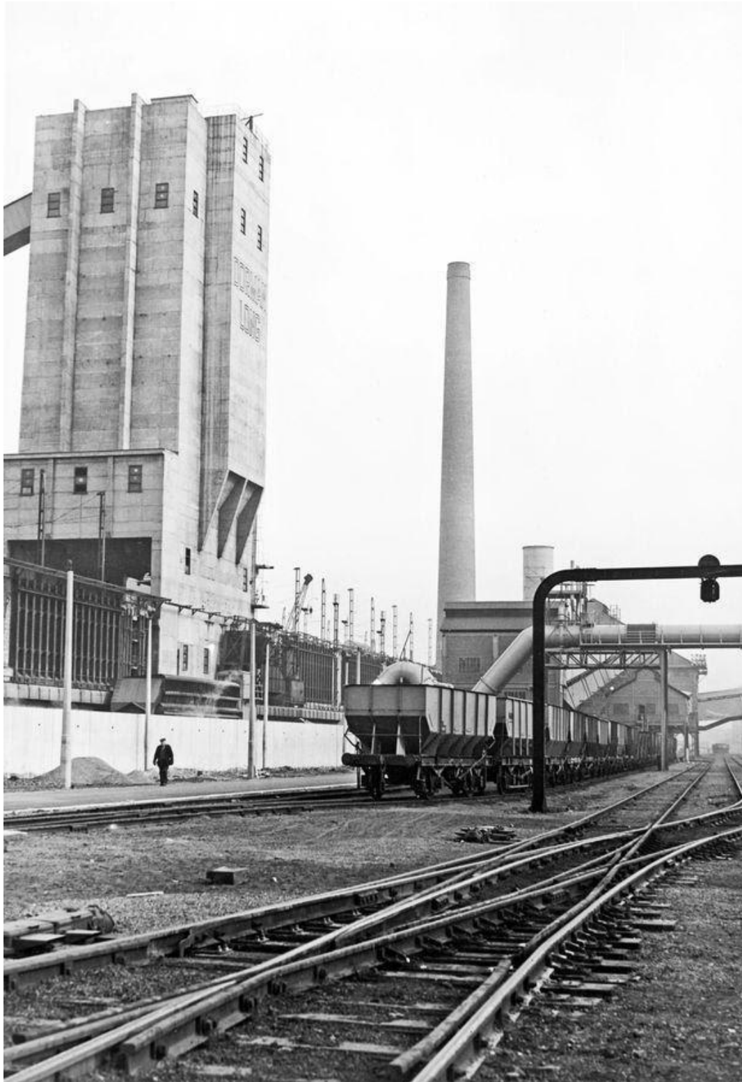
A lone worker is dwarfed by the 'Dorman Long Tower' © Teesside Archives, British Steel Collection.
