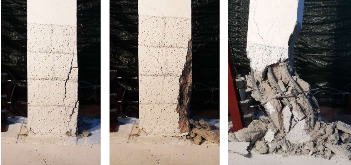
Fig. 8. Evolution of damage in the control cantilever.
