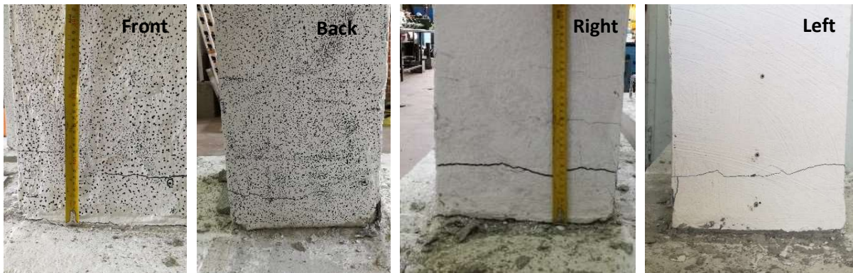
Fig. 13: Damage state at the end of the test for SRG2.
