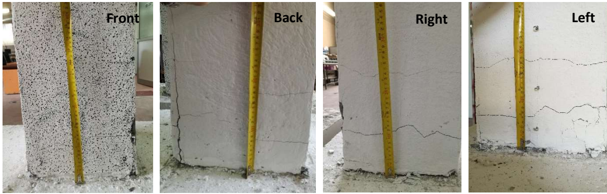
Fig. 12: Damage state at the end of the test for SRG1.
