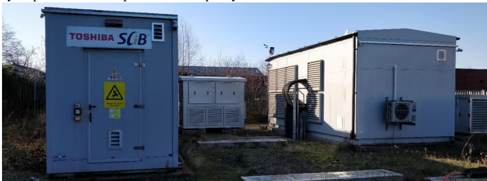
Fig. 3. Willenhall energy storage system
