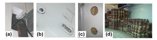
Figure 1. Fire hazards observed by insurance inspectors: (a) damage around structural steelwork and pipe and cable installation; (b) forklift truck damage to ceiling panels; (c) holes through both sides of a panel, where pipework was going to be, or had previously been, installed; (d) typical accumulation of fire load in a sandwich panel building.
