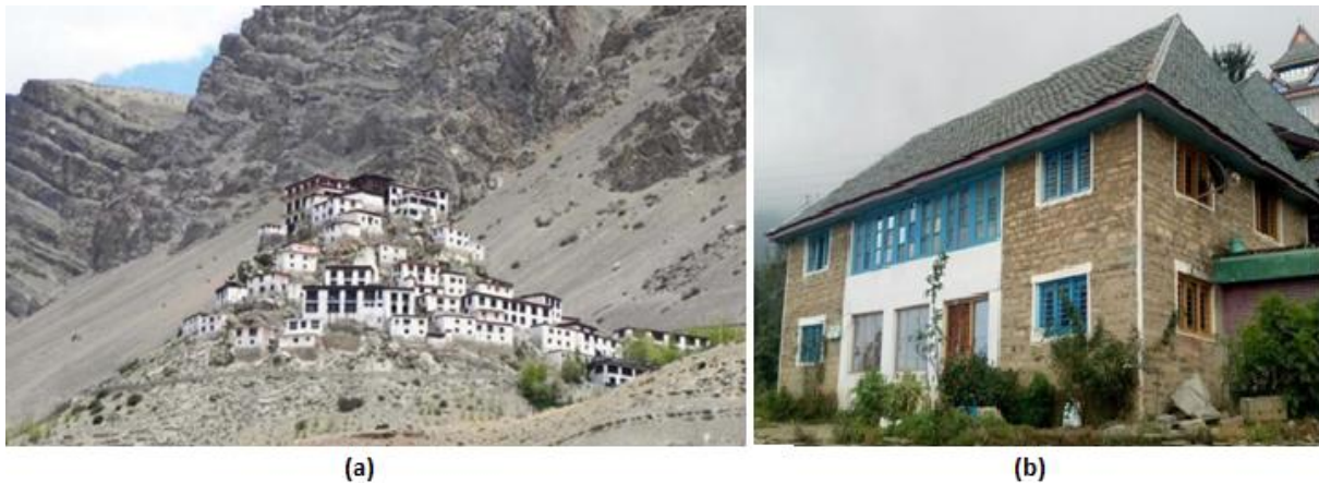
Fig 1: a Kii monastery in village Kii in Lahaul and Spiti district of Himachal Pradesh (Sood et al. 2012), b typical stone masonry house with sloping roof in Himachal Pradesh
