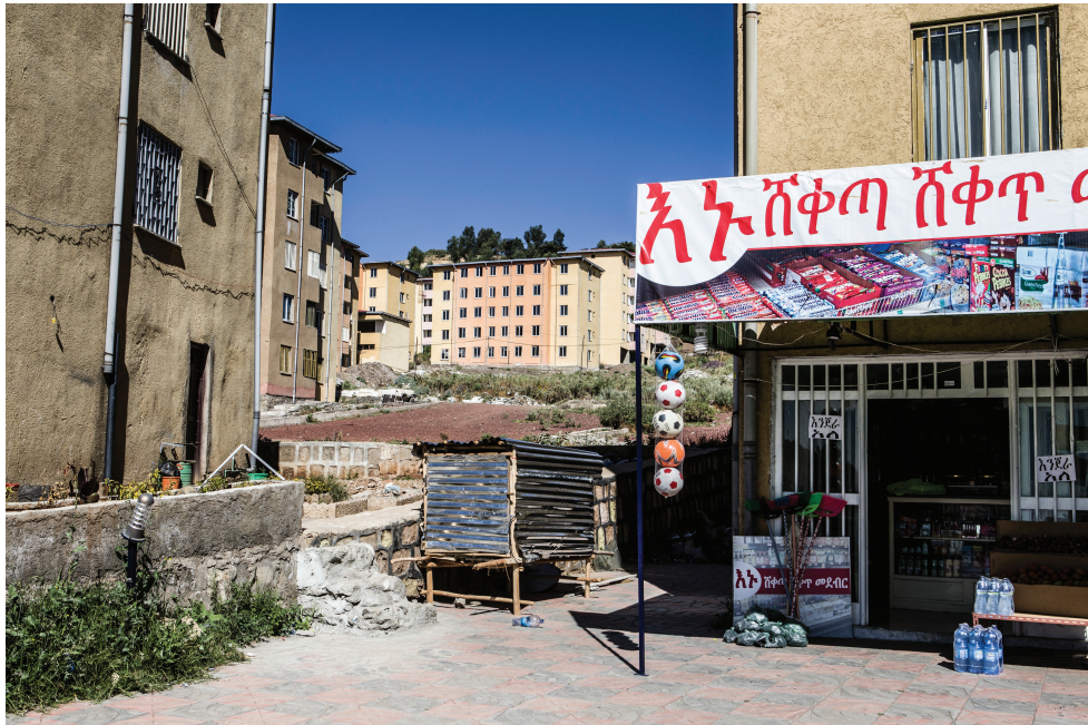
FIGURE 4 Retail space in Yeka Abado (photo © Mark Lewis)
