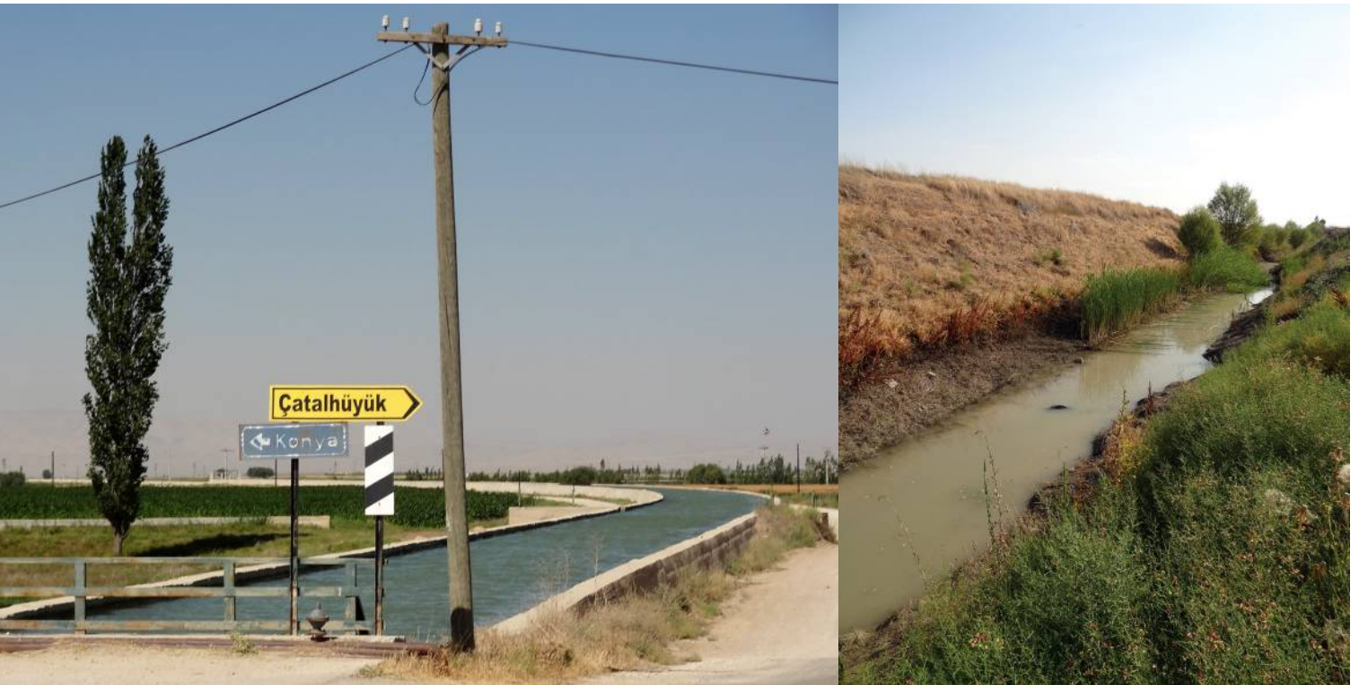
Figure 2. Channelized water system in the modern landscape: (a) the modern Çarşamba River is confined to a concrete channel immediately adjacent to the site; and (b) a deep irrigation ditch to the south of the site used to provide water to surrounding fields (via pumps and the concrete channels seen in fig. 1).
