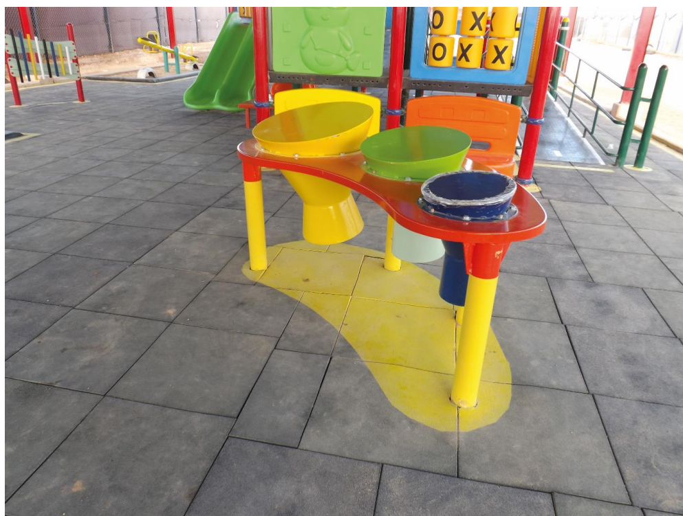
Figure 15: New constructed space – deteriorating equipment in the Inclusive Playground
