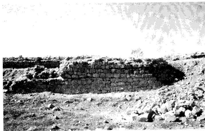
Figure 11 Achir Palace, detail of exterior wall, east side (Pb. M. Carver)
