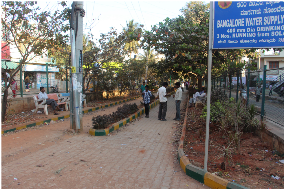
FIGURE 5 The pipeline is made visible as a political project of water provision in Soladevanahalli (photo by Vanesa Castán Broto)
