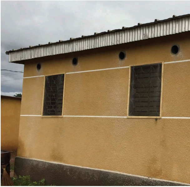
Fig. 1. An example of the SET innovation that includes closing points of entry for mosquitoes into the home (e.g., closing eaves in houses where they remain open), adding mosquito barriers to windows and doors (e.g., installing window screening), installing tubes into the eaves, and placing an insert with insecticide into the tubes.
