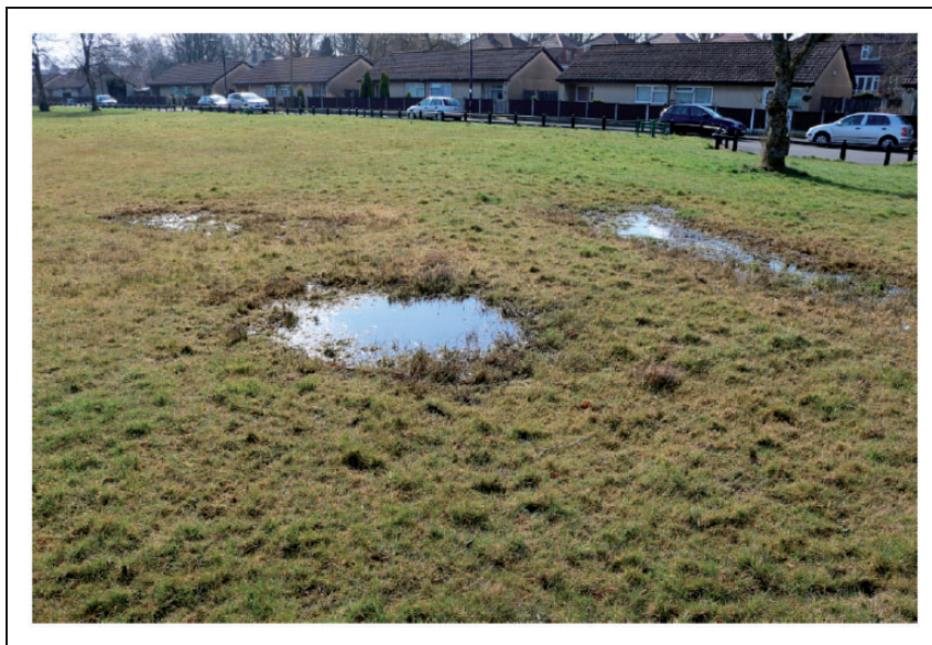
Figure 7. Subsidence and waterlogging along the brook's course.
