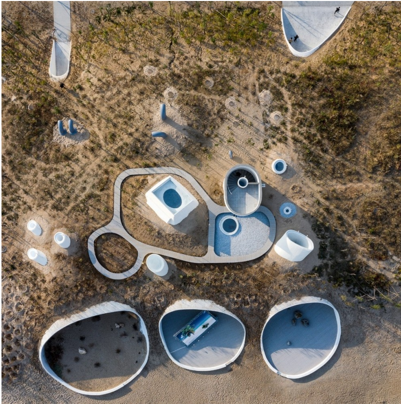
Figure 1 UCCA Dune Art Museum, bird eye of the building which is hidden in the existing sand of the seaside site.
