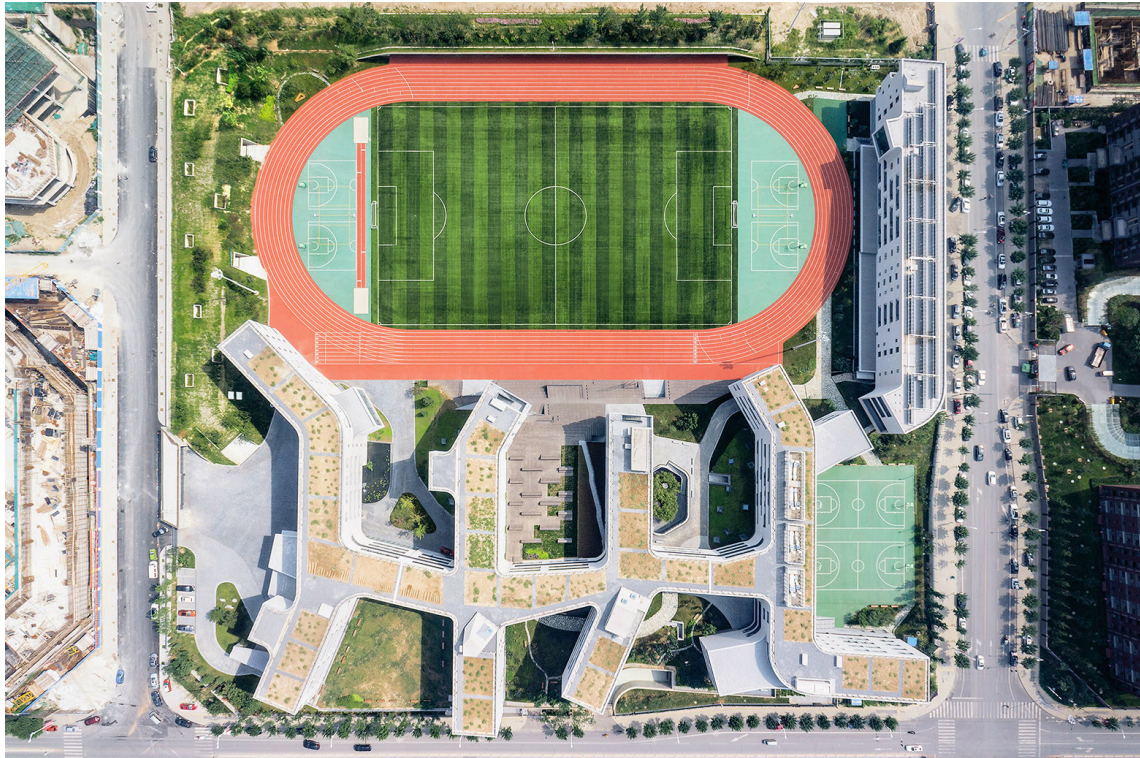
Figure 5 Garden School, birds eye of the interconnecting campus buildings and interweaving landscapes.
