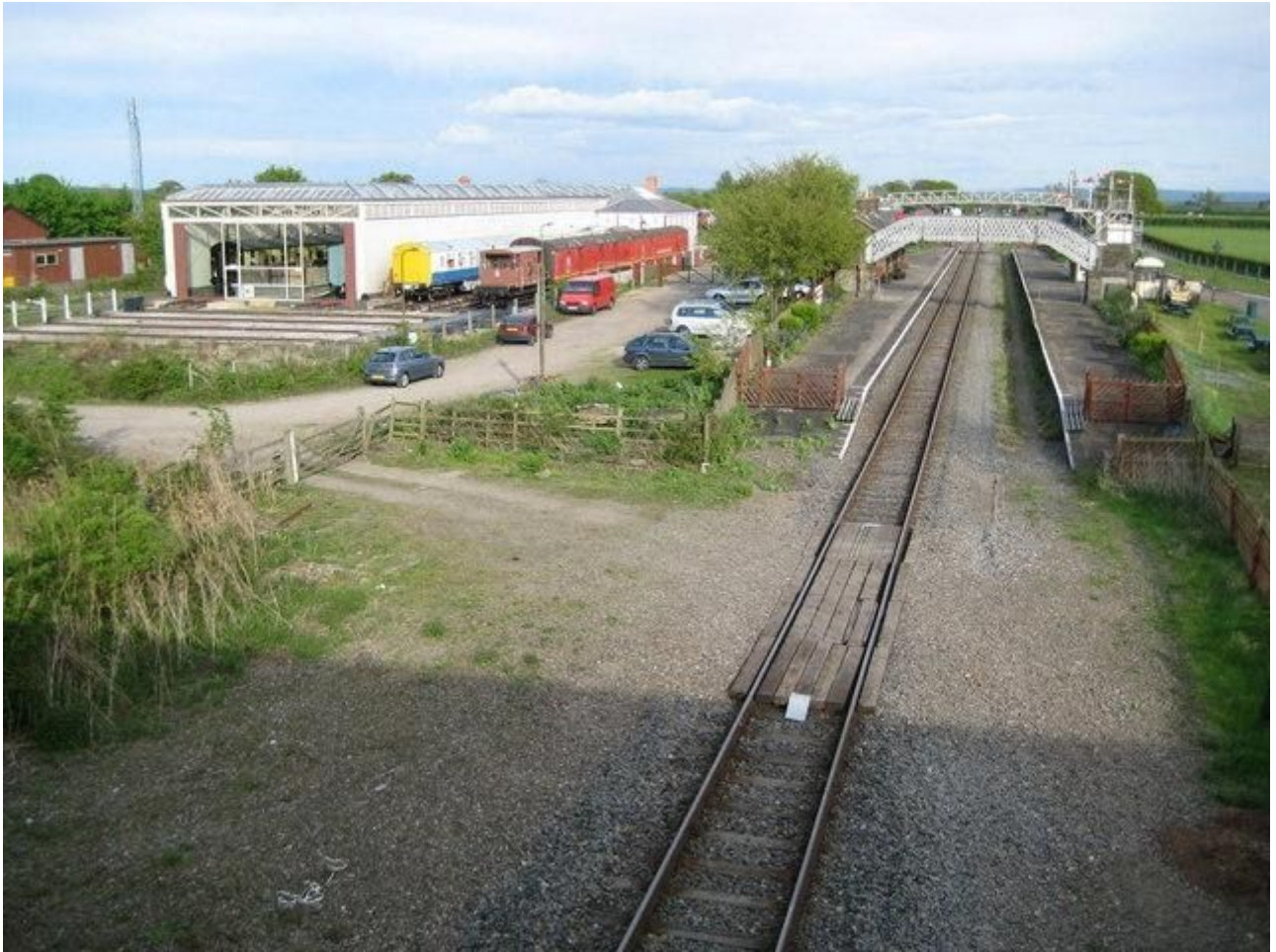
Figure 11: Quinton Road Station, the end of the line and subject of the closing scenes of Metro-land. This image was taken from the Geograph project collection. The copyright on this image is owned by Nigel Cox and is licensed for reuse under the Creative Commons Attribution-ShareAlike 2.0 license.
