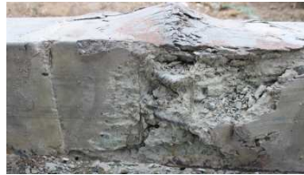
(e) Concrete crushing (TRC-0.6-0)
