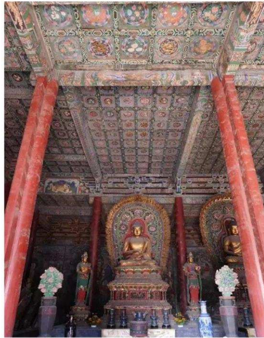
Main hall with the flat suspended ceiling.
