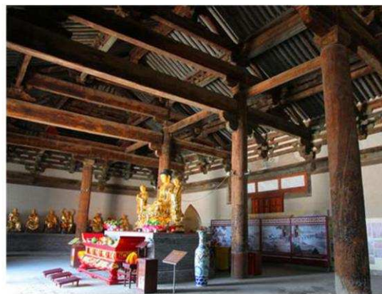
Main hall without the flat suspended ceiling.
