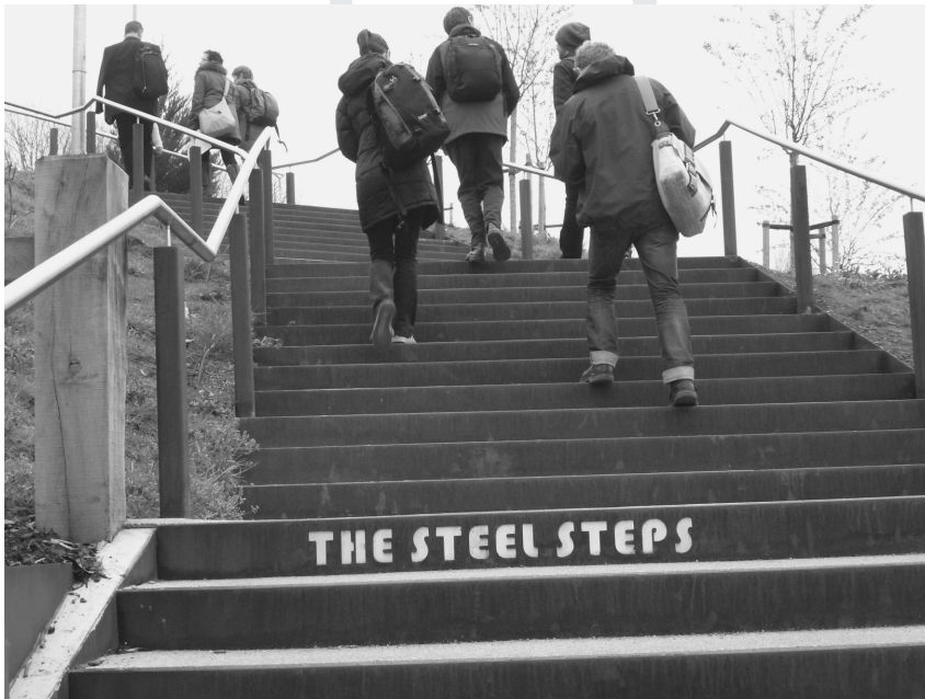
FIGURE 13.4 South Street Park: the Steel Steps.
