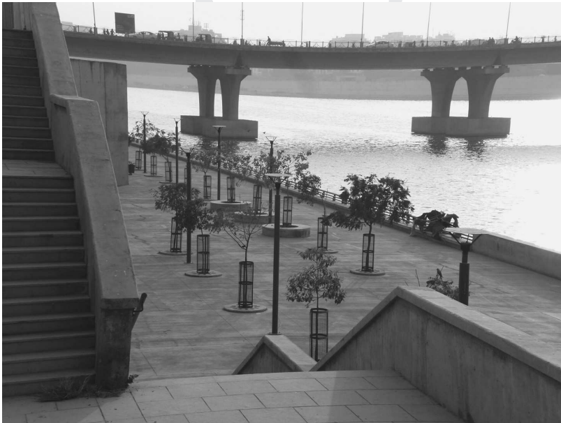
FIGURE 13.6 The Riverfront Park (upper level) is visually disconnected from the river (lower level), and physical access is made at few entry points.
