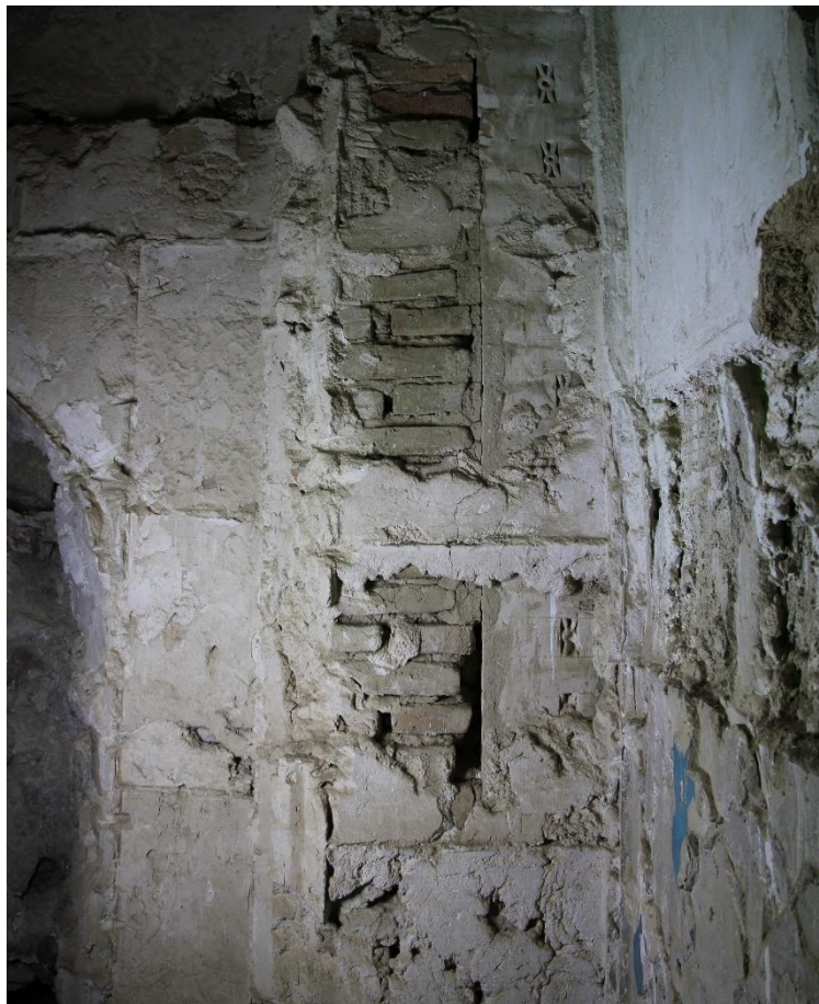
Figure 3: Construction break on the right of the mihrab
