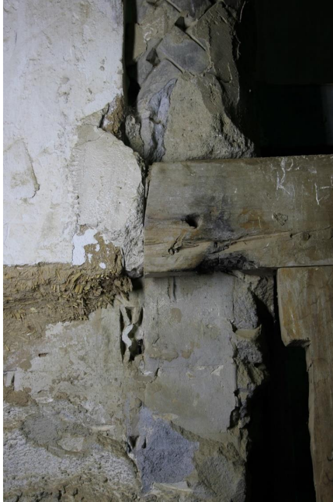
Figure 6: Corner to the right of the mihrab recess; detail of the original brickwork and later column
