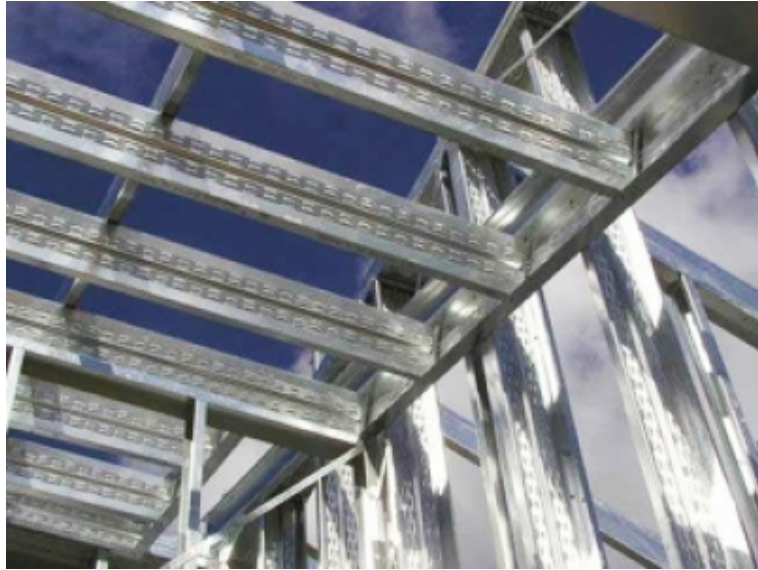
Fig. 3. Application of slotted perforated CFS beams
