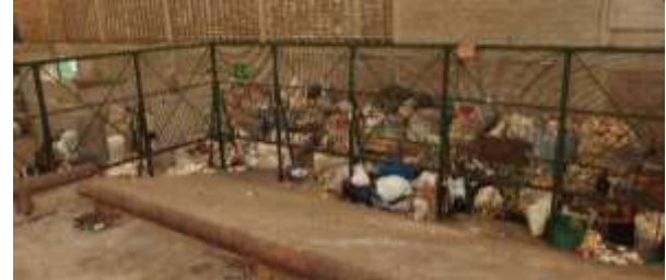
Figure 2. CL MRF – view from truck unloading area down slope, to grate and warehouse floor.
