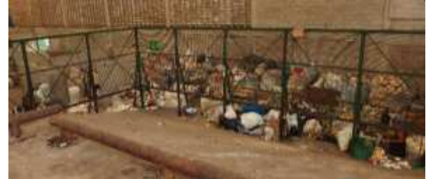
Figure 2. CL MRF – view from truck unloading area down slope, to grate and warehouse floor.
