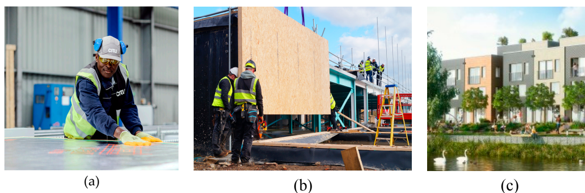
Figure 7. Case study 3 construction phases of the pioneering sustainable development (credited to CITU [43]). (a) components production in factory, (b) site assembling, (c) final view.
