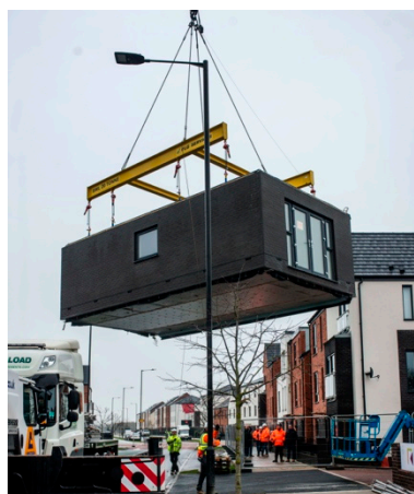
Figure 4. Case study 1 installation of prefab modules (credited to Ilke Homes).
