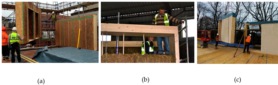
Figure 8. Case study 4 timber-framed panels insulated with straw bale (credited to Modcell). (a) wall installation, (b) straw filling, (c) on site installation and waterproofing.
