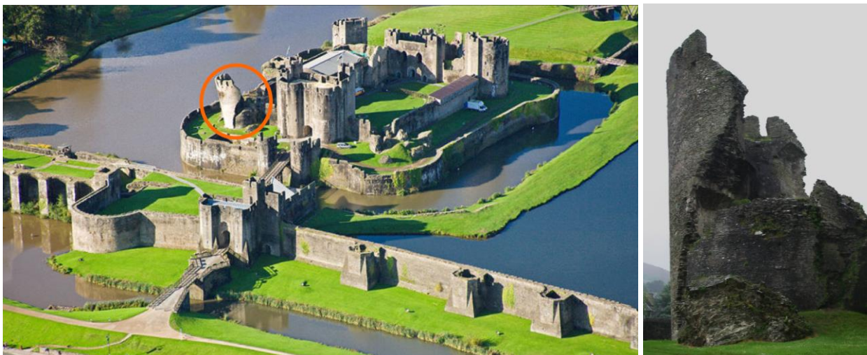
Figure 1. Southwest leaning tower of Caerphilly castle. The red circle indicates the location of the southwest leaning tower.
