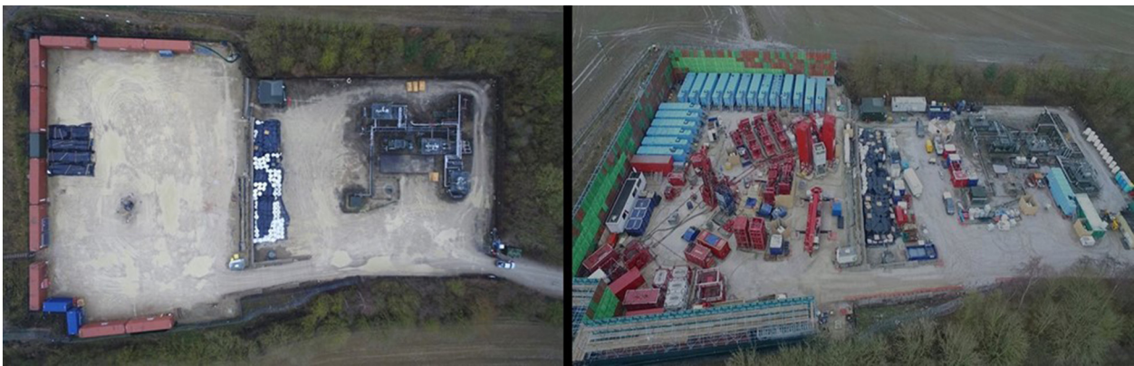
Fig. 6. Images of the Third Energy Kirby Misperton well site in December 2017 (left hand side) and April 2018 (right hand side), illustrating the extra equipment brought onto the site in preparation for shale gas extraction. (Credit: Eddie Thornton).
